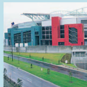
Colonial Stadium - Melbourne
