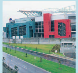
Colonial Stadium - Melbourne
