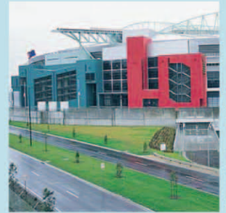
Colonial Stadium - Melbourne
