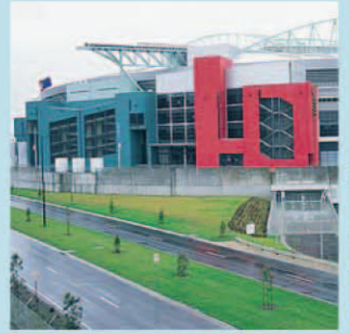
Colonial Stadium - Melbourne
